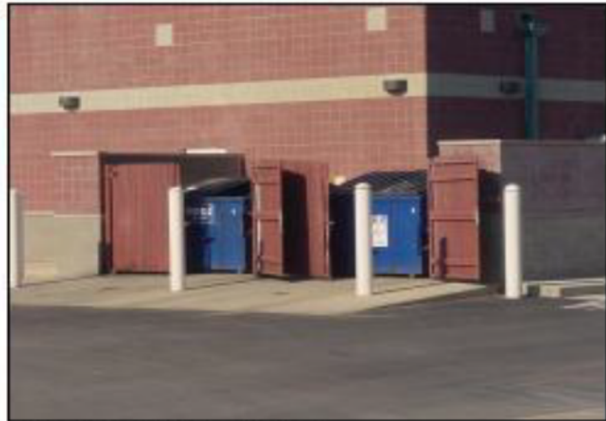
Figure 2-14 Screened Refuse Area
