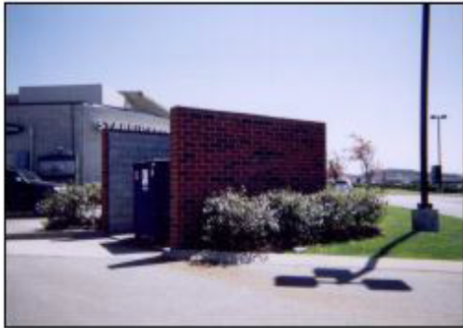
Figure 2-13 Screened Refuse Area
